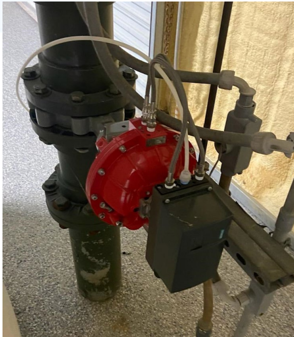
New Plant Control Valves
